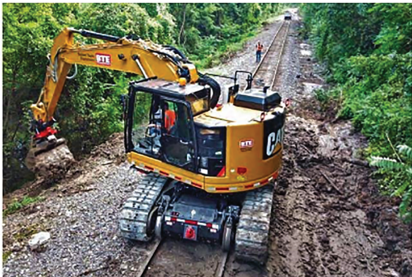
For this muddy disaster, BTE supplied Greis Trucking & Excavating with the hi-rail excavators to get the mud and debris removed from the track and to help repair flooded damage ditches.
